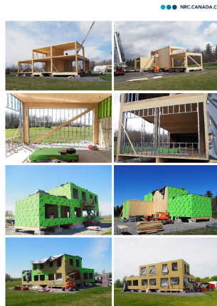
Figure 3. Photographs of mass timber test structure during construction.
